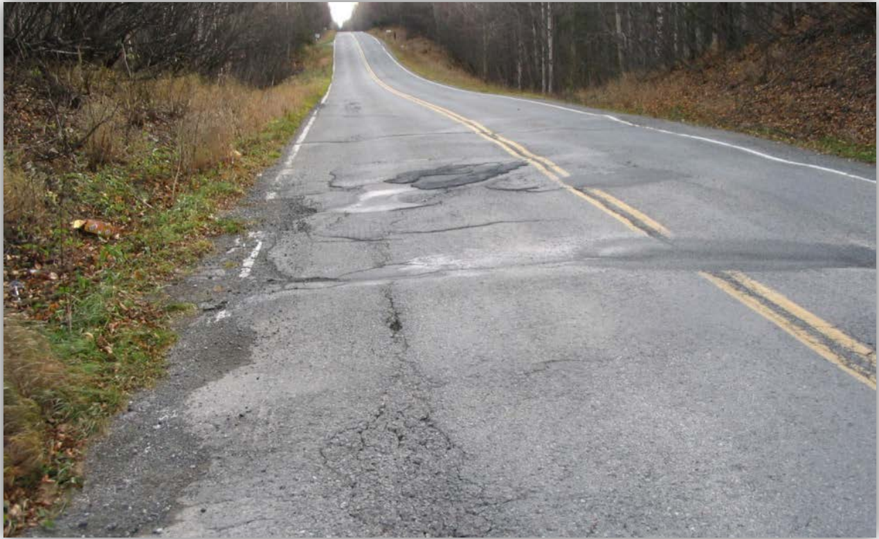
Figure 1.4 West Dimond Boulevard Showing Pavement Deterioration
