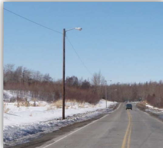
Figure 3.7 Roadway Illumination Pole
