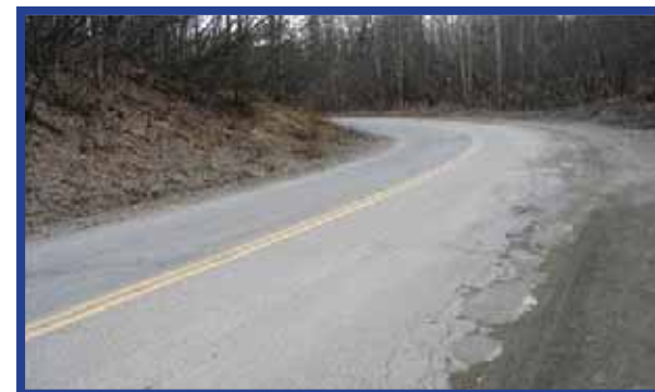
LACK OF LIGHTING, LANDSCAPING, PAVED SHOULDERS & POOR SIGHT DISTANCES
