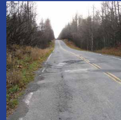
SUBSTANDARD ROAD FOUNDATION & SURFACE
