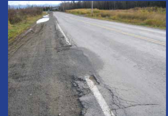
SUBSTANDARD ROAD FOUNDATION & SURFACE
