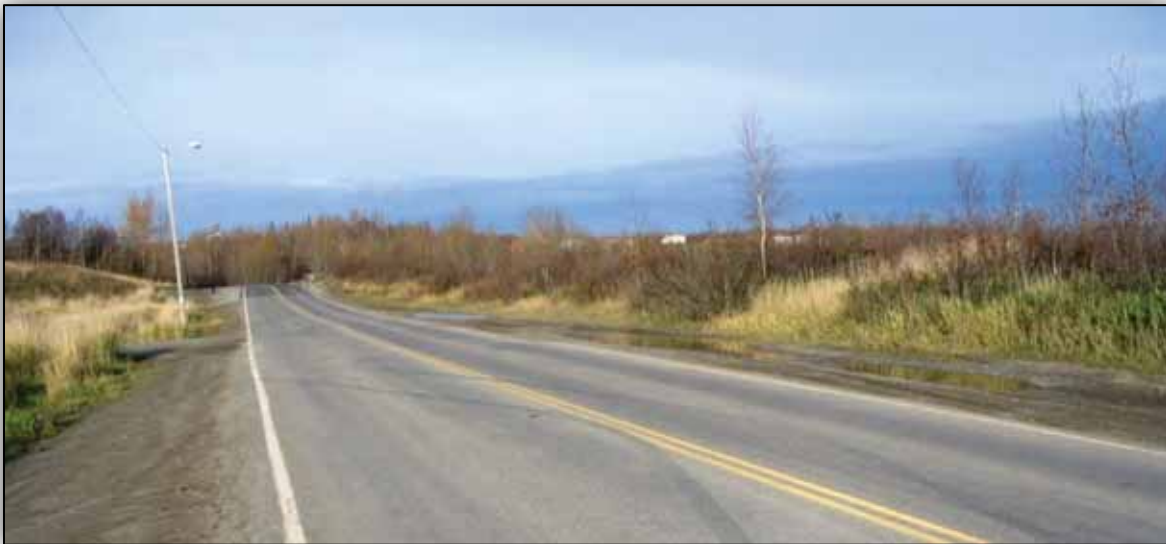
Figure 3.1 West Dimond Boulevard between Westpark Drive and Sand Lake Road
