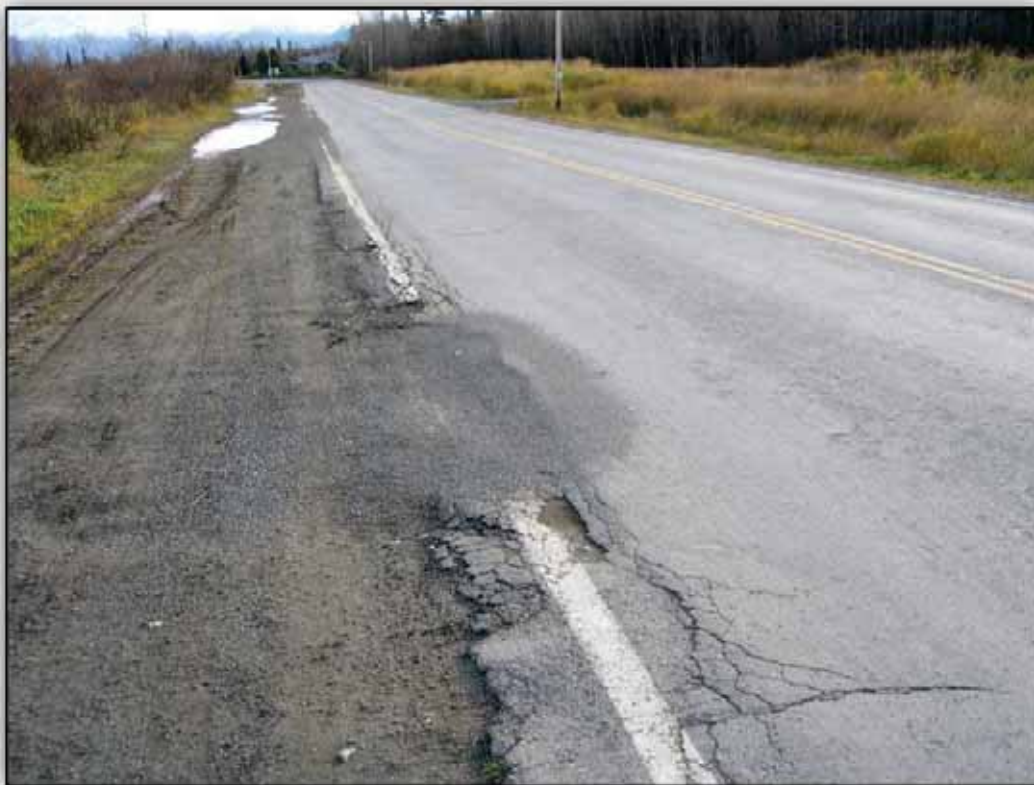
Figure 1.4 West Dimond Boulevard Pavement Deterioration
