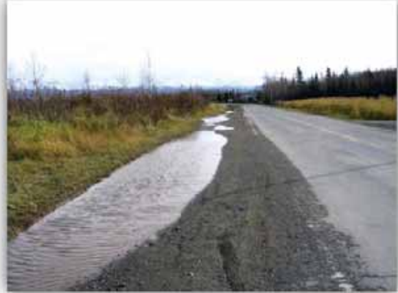
Figure 3.6 Ponding During Summer
