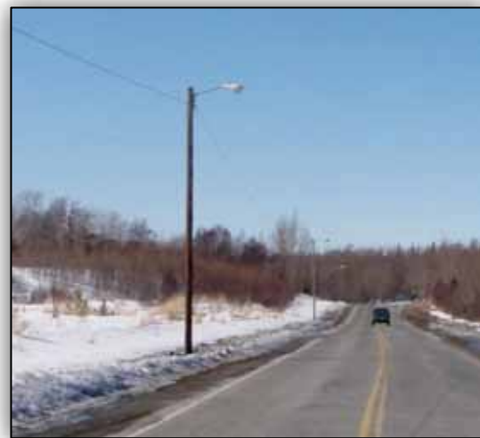
Figure 3.7 Existing Roadway Illumination Poles
